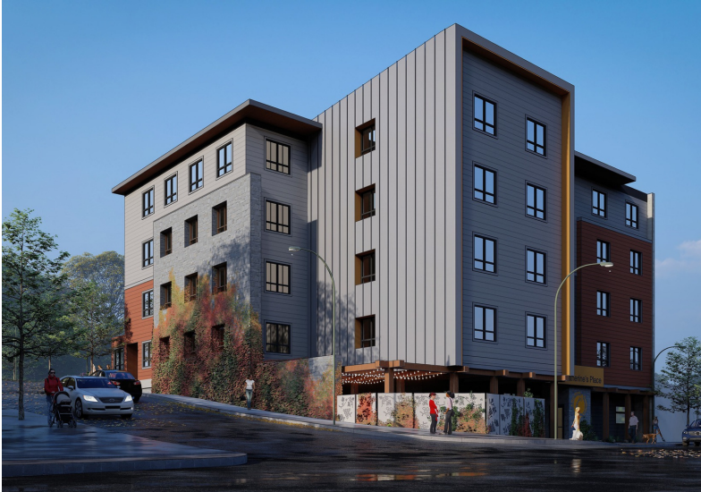
Katherine's Place - under construction at 562 Tranquille Rd.
